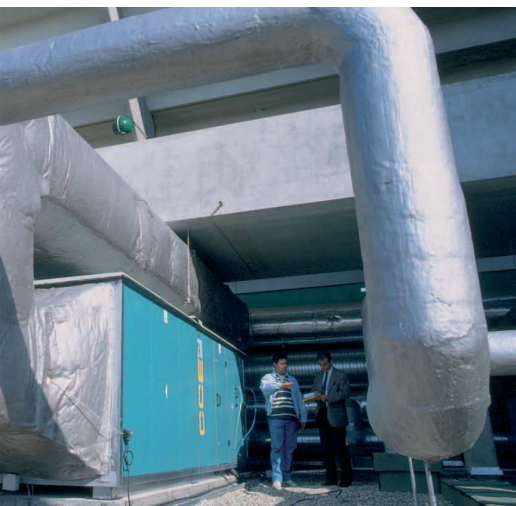
Circulating pumps for building management
